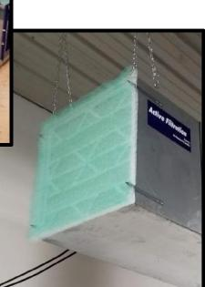
Active Filtration units can be configured with a pre-filter pad. The benefit of this light and inexpensive low MERV rating filter is providing lengthened filter life. The pre-filters are particularly great for areas that deal with a lot of large particles like sawdust and general dust.
